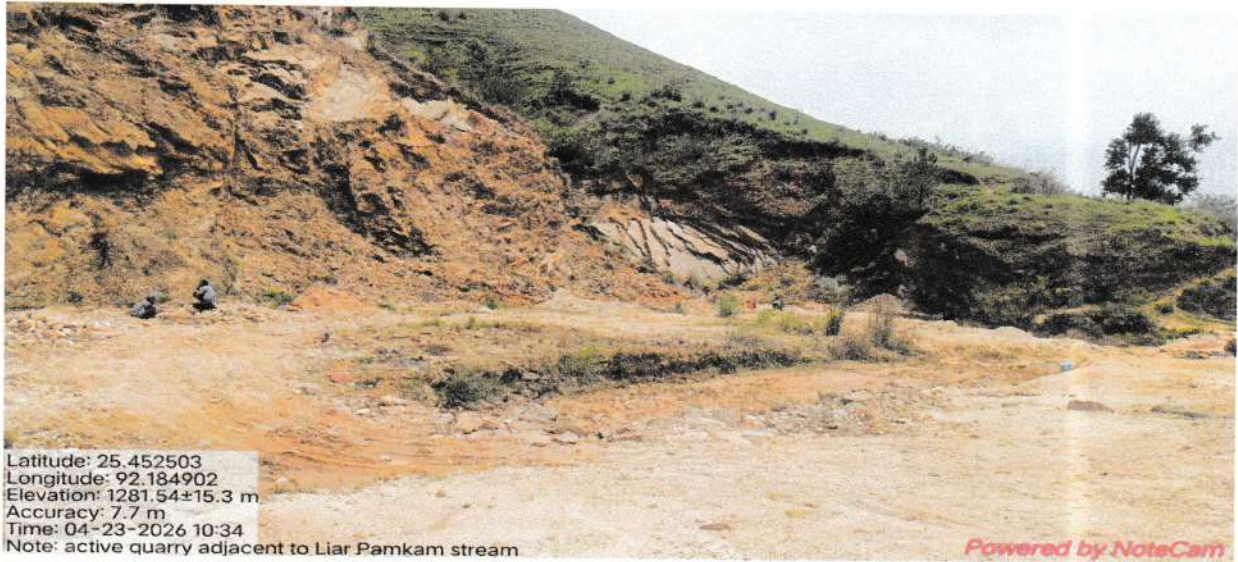
ACTIVE PRIVATE QUARRY ADJACENT TO LIAR PAMKAM STREAM BY THE OUTSKIRT OF MYNTDU RIVER
